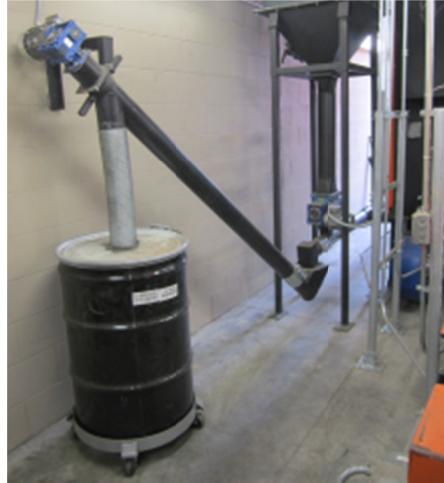
Figure 9 – Automated Ash Collection from Pellet/Chip Boiler
