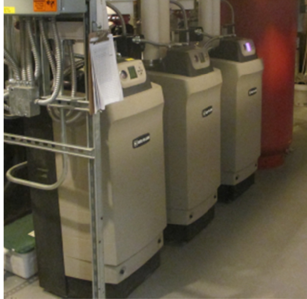
Figure 2 – Weil McLain Ultra Boilers
