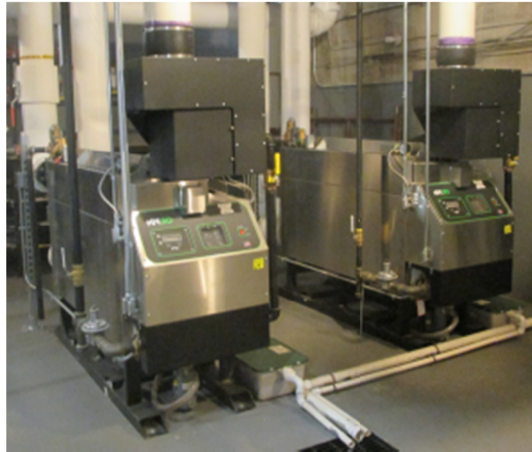
Figure 1 – KN-30 Propane Boilers
