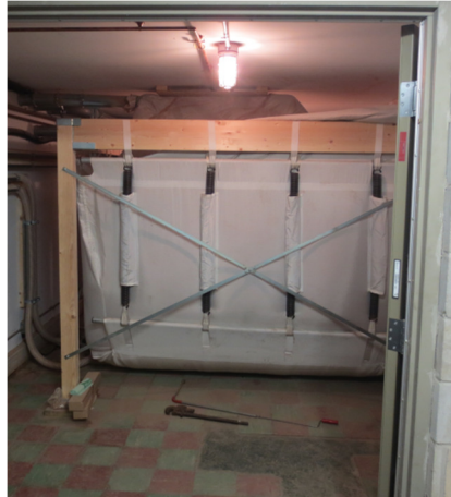
Figure 7 – Indoor Pellet Storage
