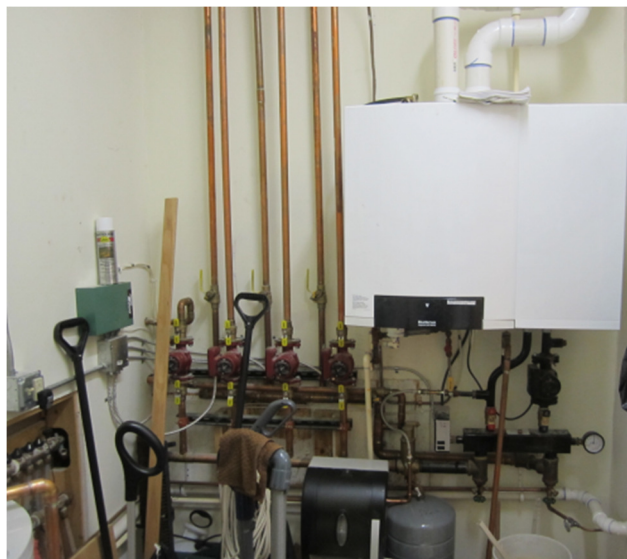
Figure 3 – Boiler and Hydronic Distribution
