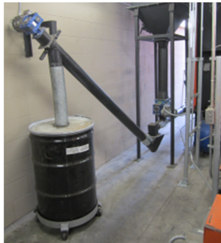
Figure 8 – Automated Ash Collection from Chip Boiler
