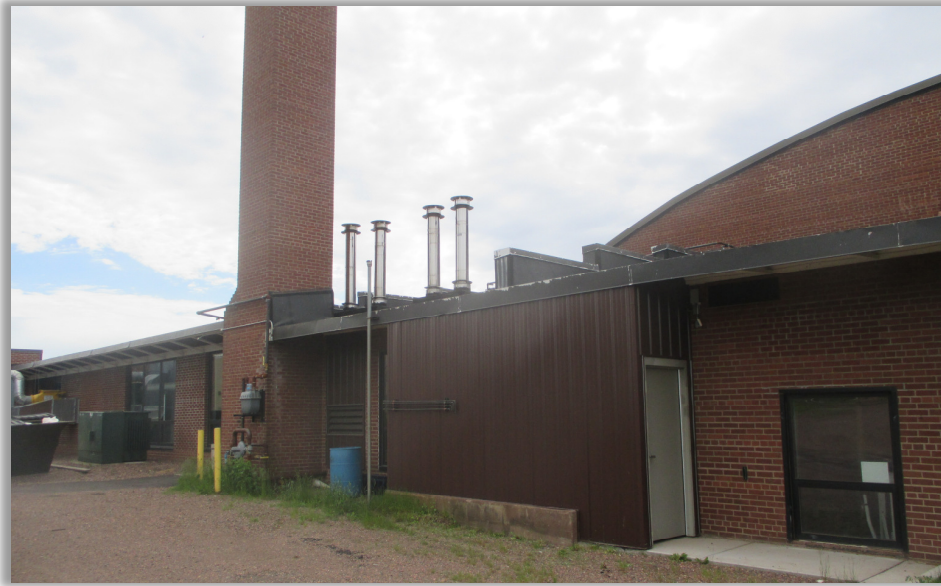
Figure 1 – Central Boiler Room
