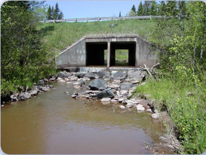
Upstream view of perched culverts
