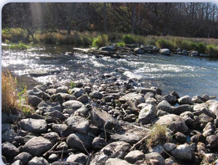
Constructed riffle
