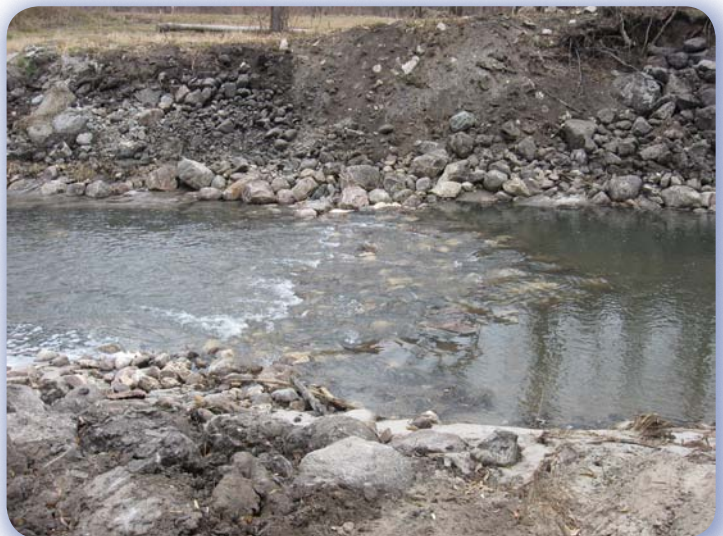
Riffle grade control
