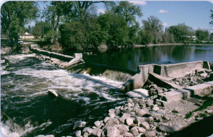
Upstream view of failed dam showing eroded left embankment and breach near right bank
