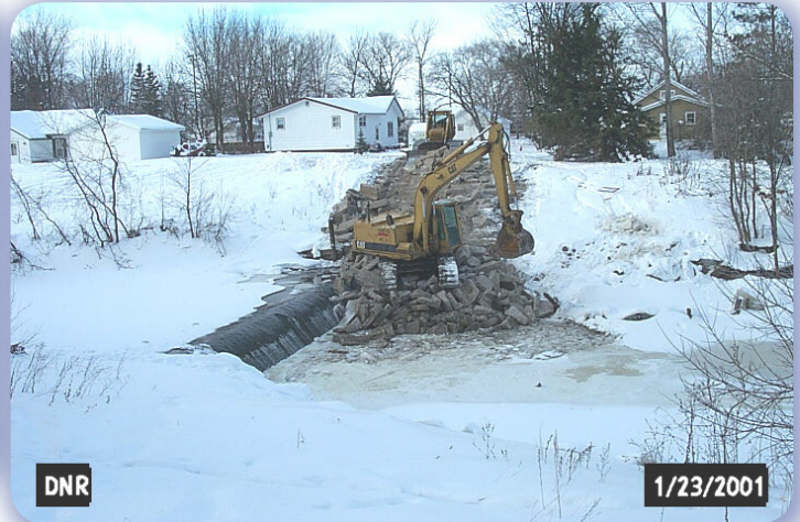
Construction of rapids base
