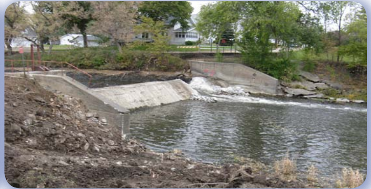
Upstream view of dam showing notch to lower pool during construction
