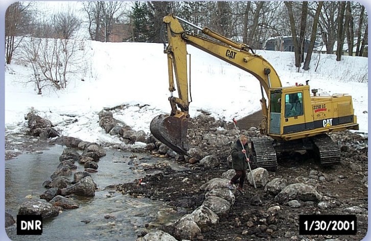
Construction of weirs
