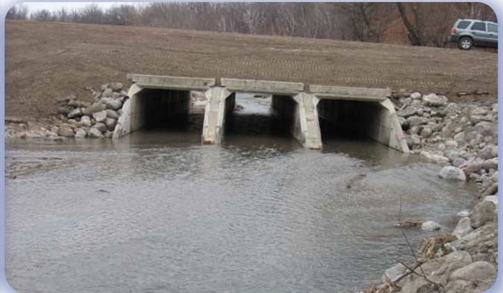
Upstream view of reset culverts
