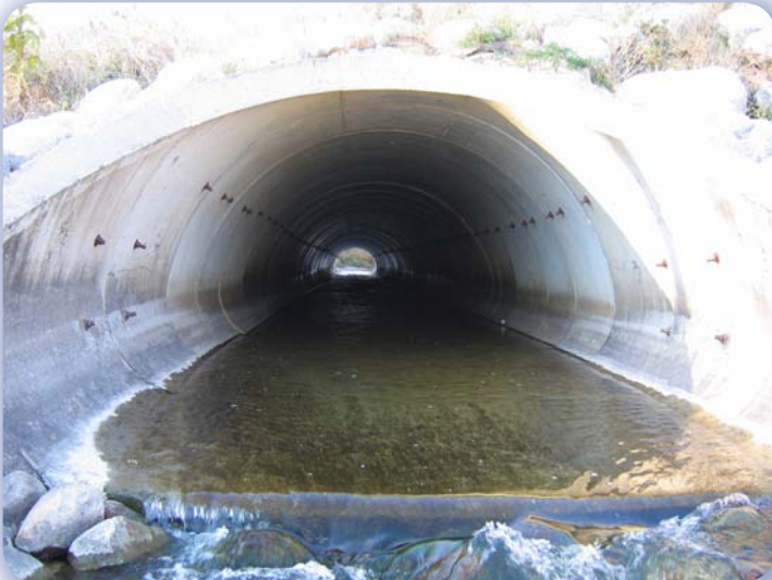
Lowest perched culvert as a barrier to fish passage
