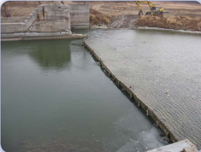
Sideview of dam showing sheet piling crest
