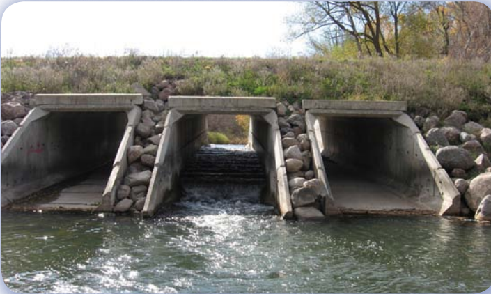
Upstream view of perched culverts
