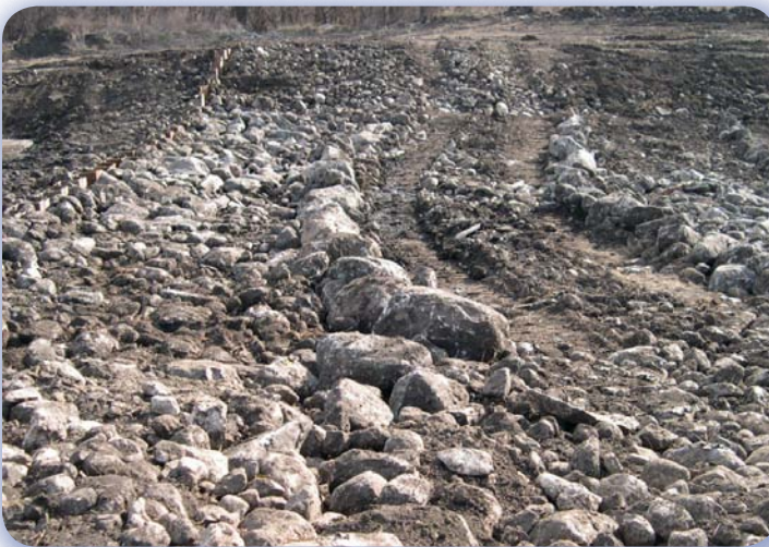
Constructed rock ramp base
