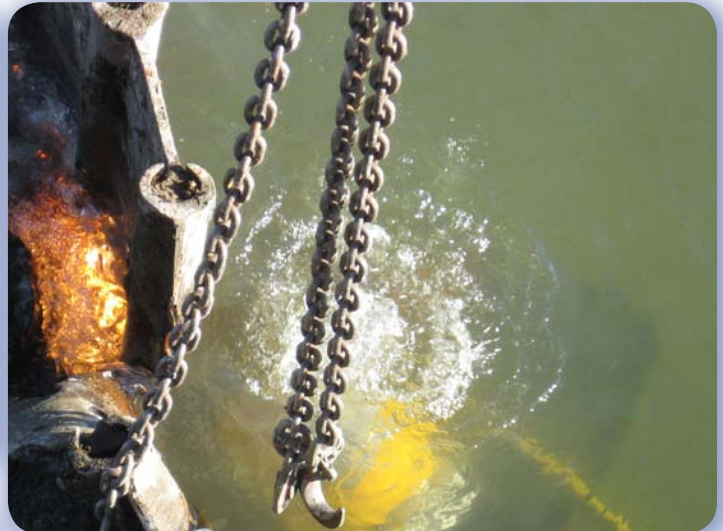
Divers cutting sheet piling
