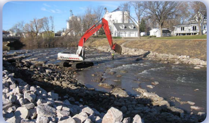
Construction of weirs in rapids
