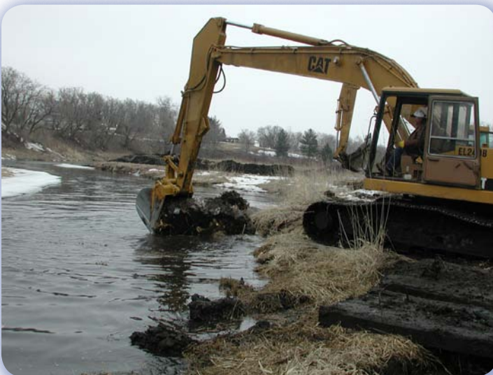
Driving root wad into bank
