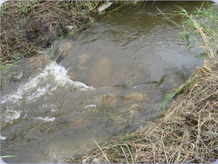
Constructed riffle
