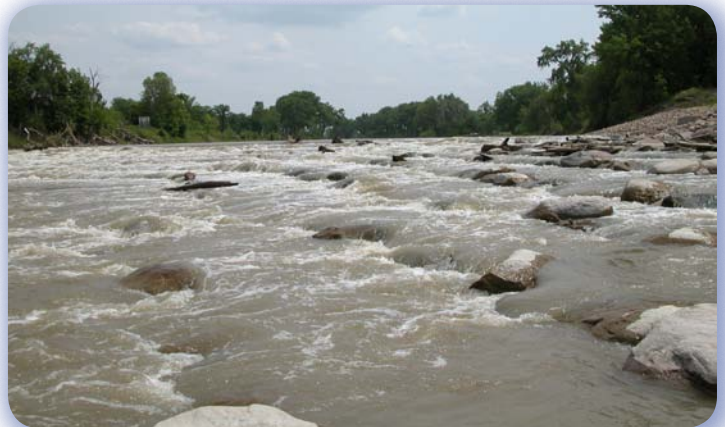
Upstream view of boulder weirs
