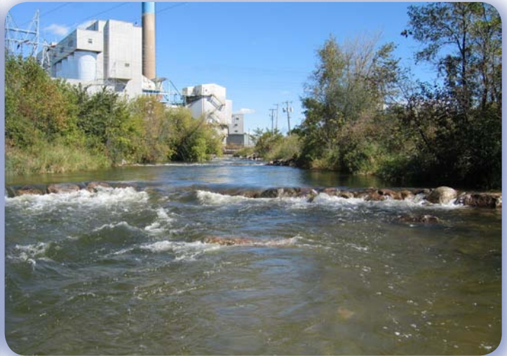
Upstream view of completed lower riffle
