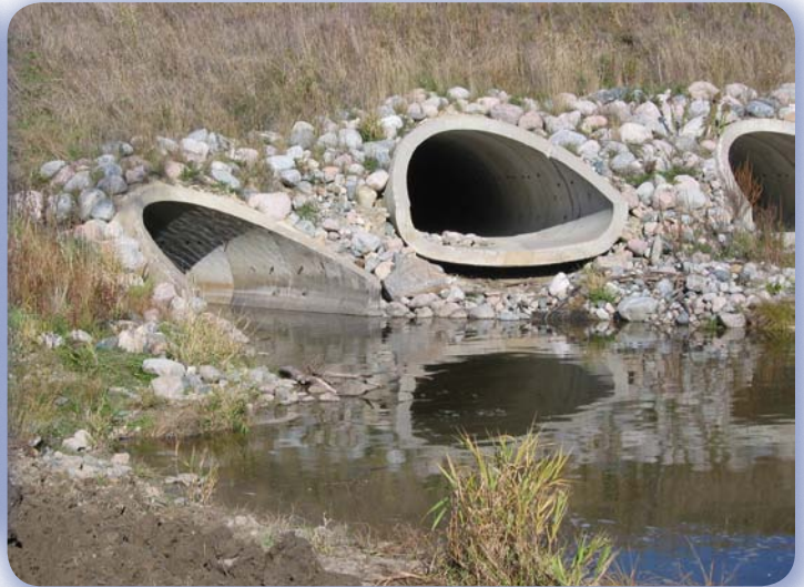
View of culverts showing tailwater pooling into lower culvert following riffle construction
