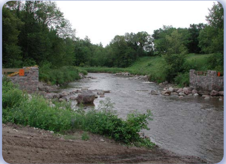
Upstream view of removed dam and completed rapids
