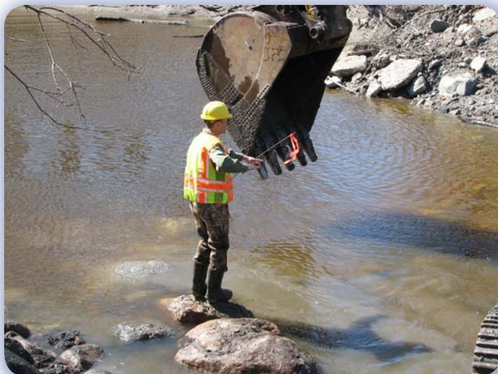
Construction of boulder weir
