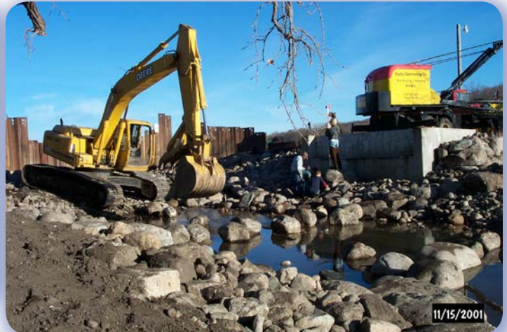
Construction of weirs
