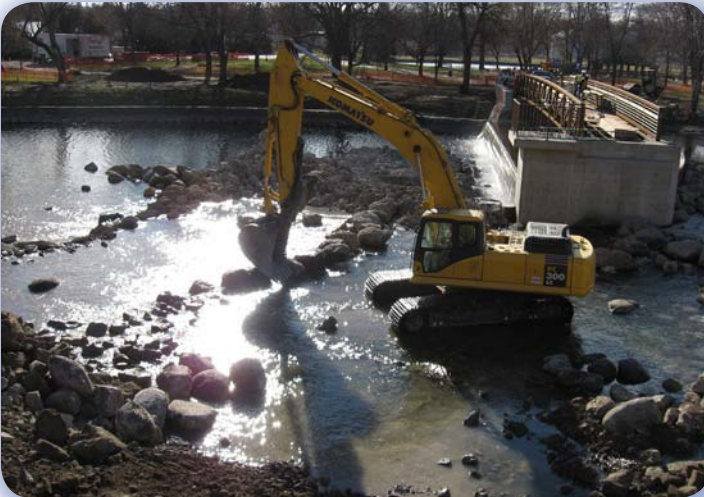
Construction of boulder weir
