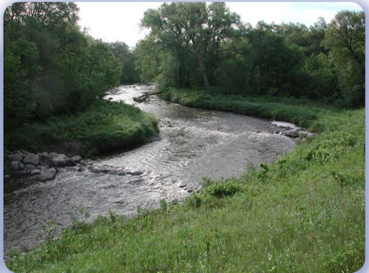
Upstream constructed riffles
