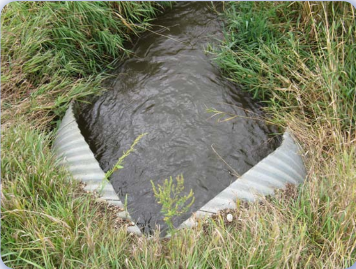
Downstream view of culvert after riffle construction. Prior to the project the culvert had over two feet of fall.
