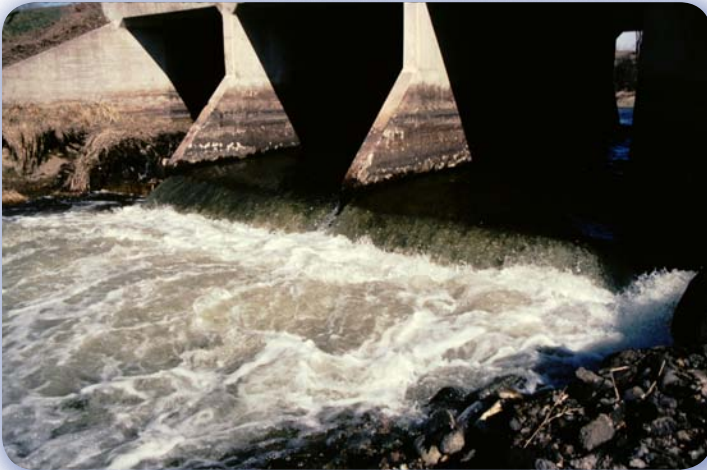
Upstream view of perched culverts
