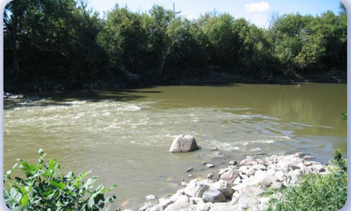
One of two downstream riffles constructed for grade control and to raise tailwater elevation below rapids
