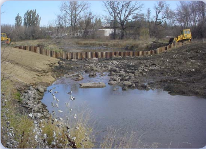
Sheet piling crest of rock ramp
