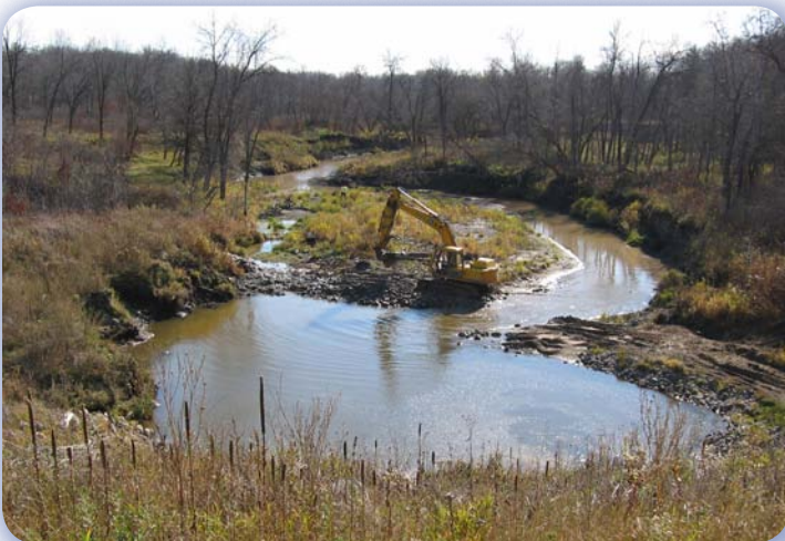
Construction of riffle
