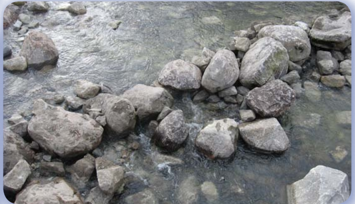
Partial weir to reduce headloss
