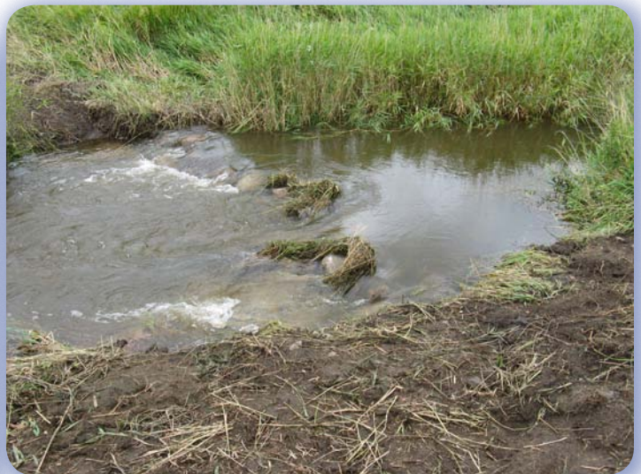
Constructed riffle
