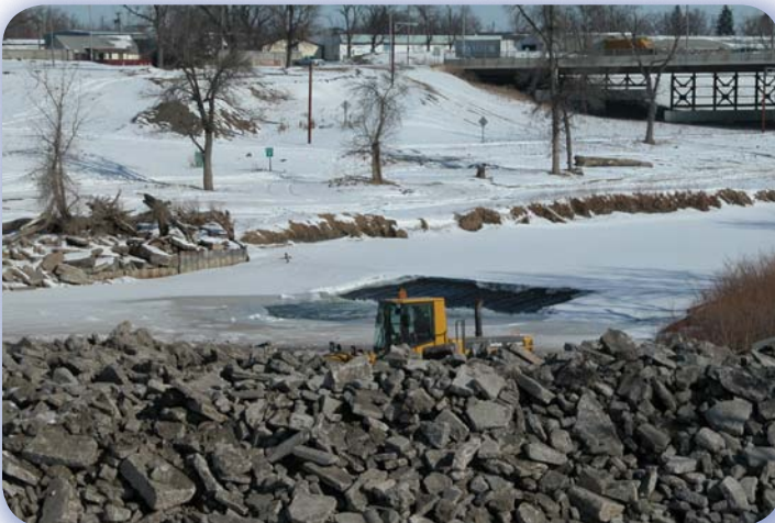
Placing waste concrete sub-base
