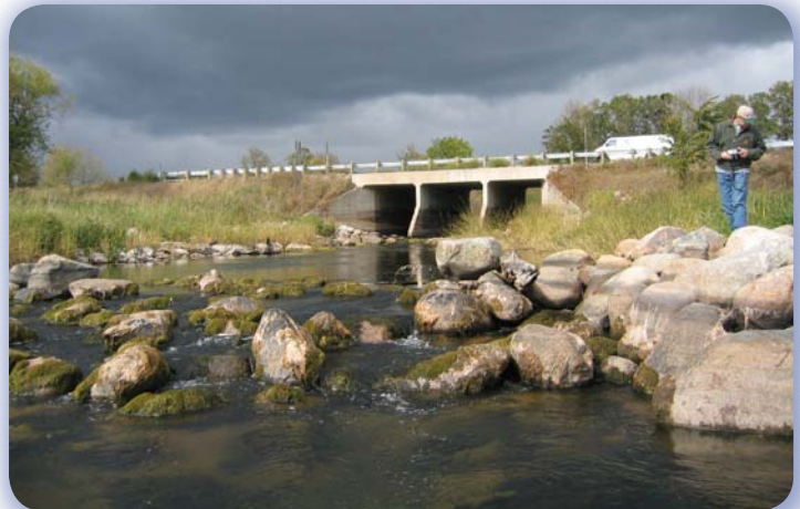
Upstream view of a riffle downstream of the culverts following river restoration in the former reservoir
