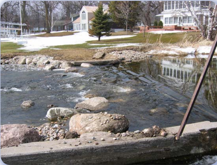
Side view of boulder weir
