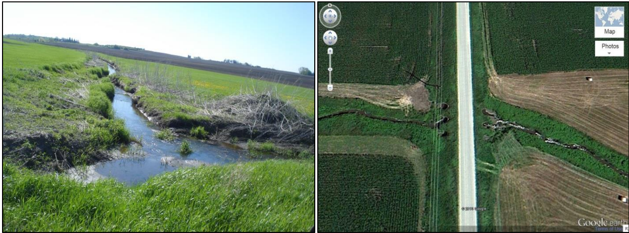
Figure 7(a) and 7(b): Identification of FFC. 1(a) standing on a roadway looking upstream at the river channel. 1(b) aerial view of the same intersection. Notice the over-widening of the perennial channel at the road intersection.
