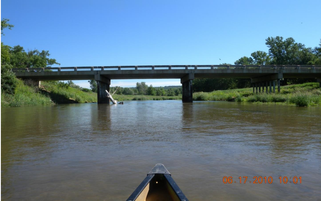
Figure 20: Photo of Beaver Creek bridge (a 'commonly found' structure on the landscape)
