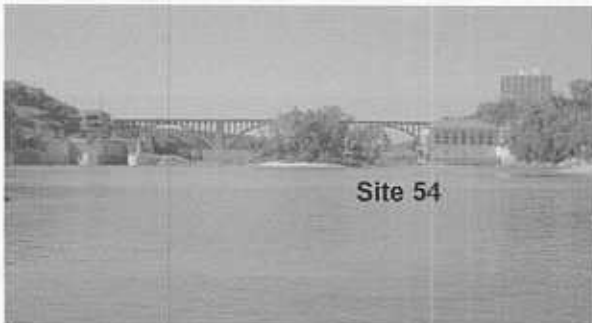
Lock and Dam 1 (Ford Dam), Site 54 is along an unnamed island and was a state listed species relocation area.
