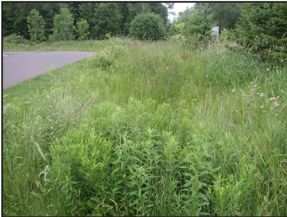
Infiltration swale with native grasses
