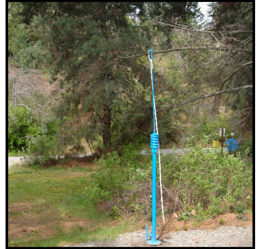
Outdoor faucet/city water source
