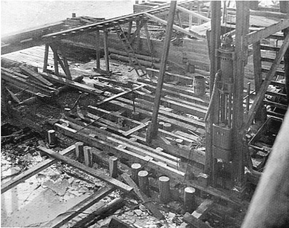
A close-up view of the steam hammer used to pound pilings during the 1916 repairs. A section of the track is shown, on its trestle across the floor of the dam.
