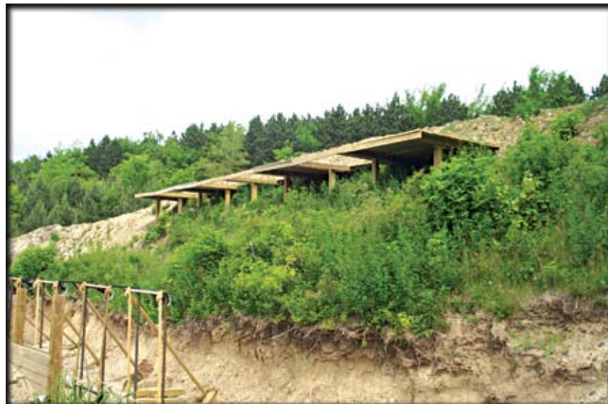
Bulletcatcher, partially constructed, using on site materials
