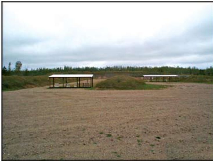
An interior berm, placed between 50 and 100 yard shooting ranges.
