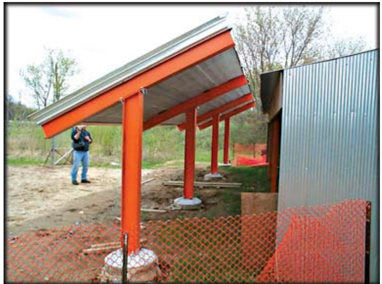
Single baffle bullet deflection
