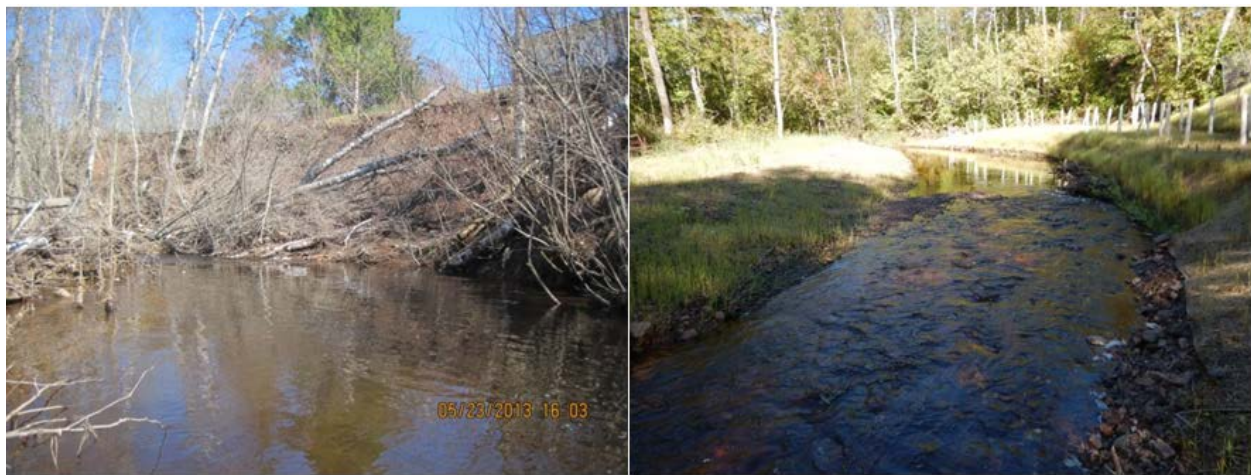
Photos: The 2015 South St. Louis SWCD bank stabilization project on East Amity Creek, upstream of Jean Duluth Road, before (left) and after (right) completion. Photo credit: South St. Louis SWCD.
