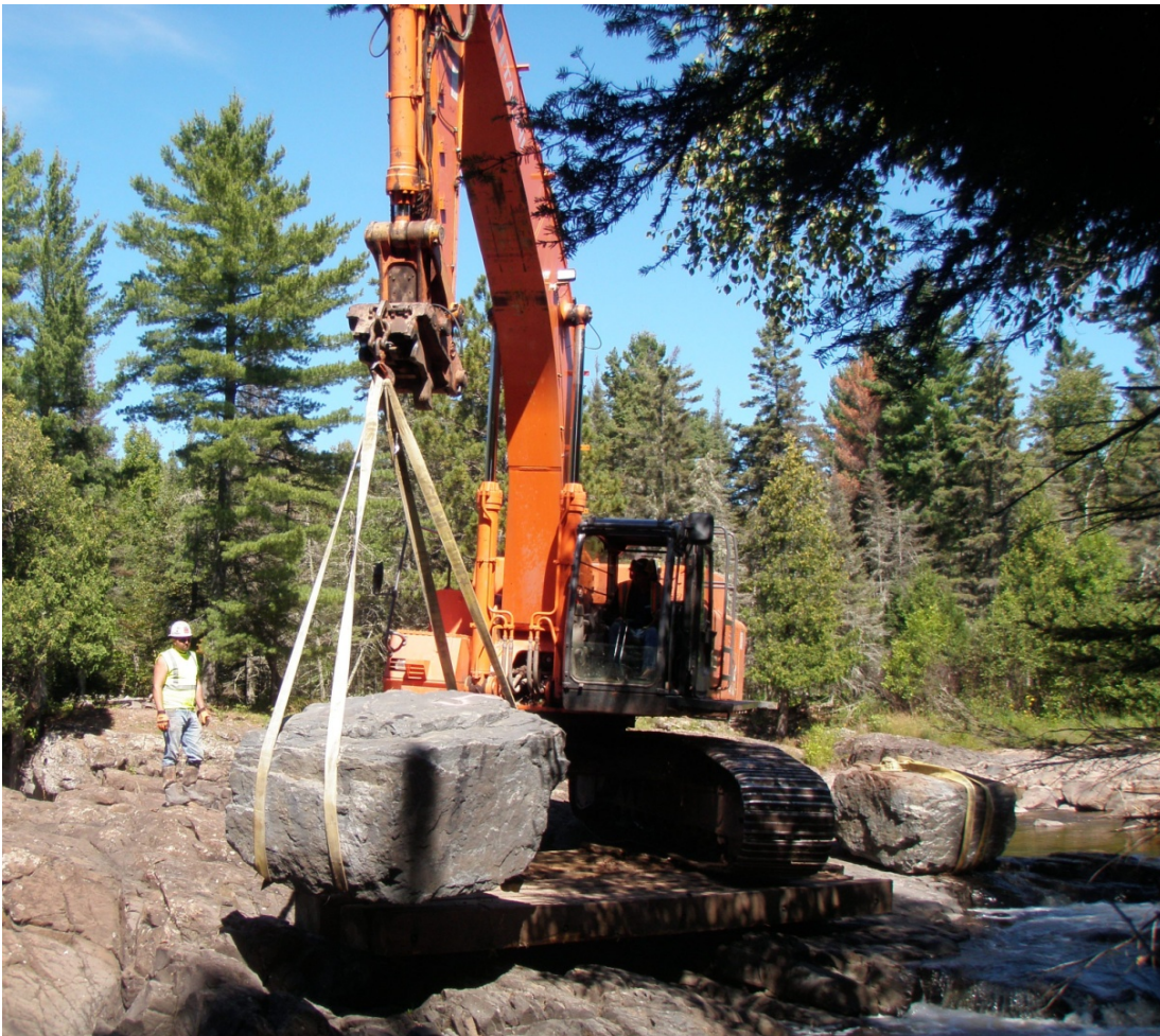
A Reuben Johnson & Son excavator operator carefully lifts one of the quarried stones for placement below the second falls on the Knife River.
