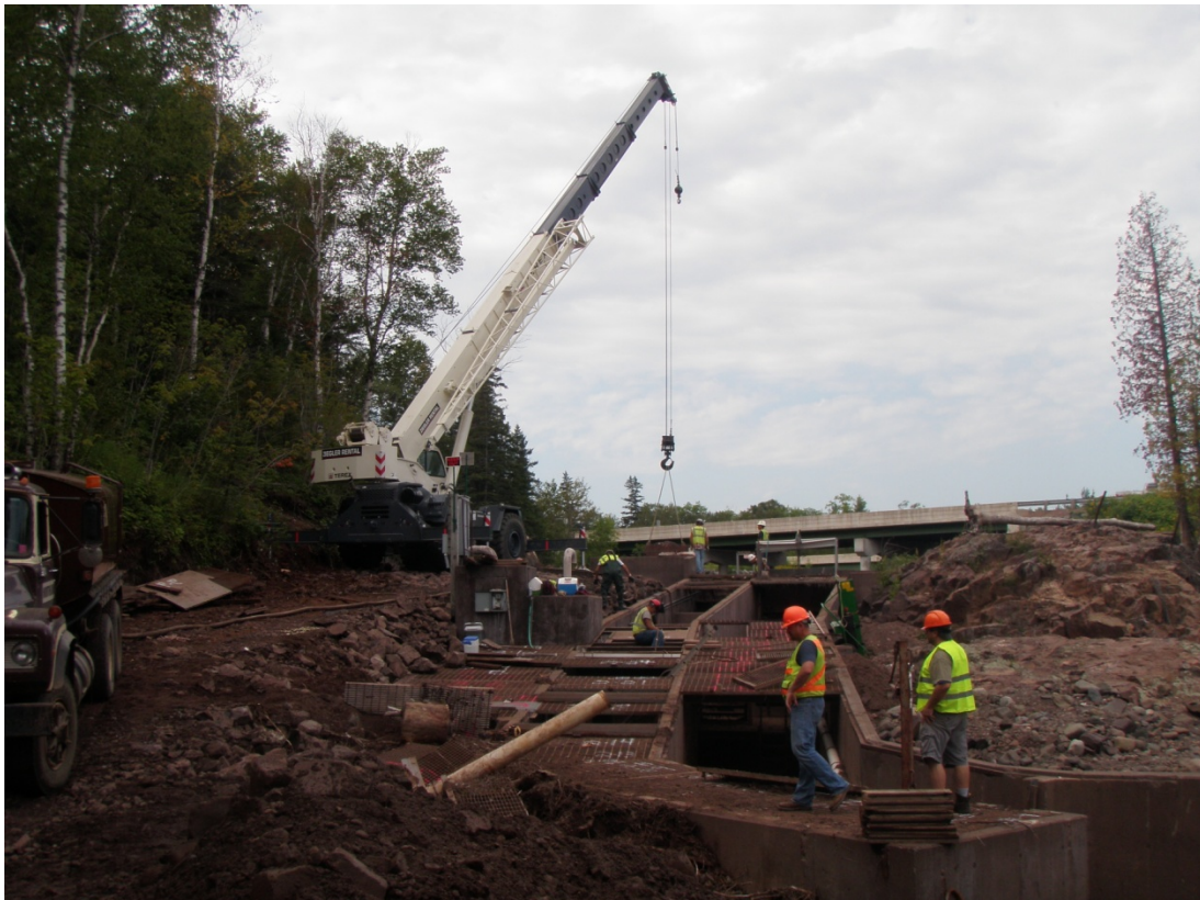
Northland Construction hard at work on the fish trap.
