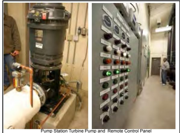
Pump Station Turbine Pump and Remote Control Panel
