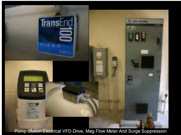
Pump Station Electrical VFD Drive, Mag Flow Meter And Surge Suppression
