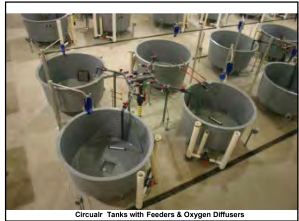
Circular Tanks with Feeders & Oxygen Diffusers
