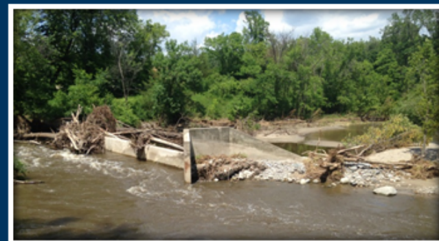
High Island Creek Dam failure
