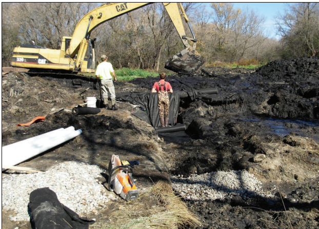
Construction work at the DNR's 1-acre lot, October 2010
