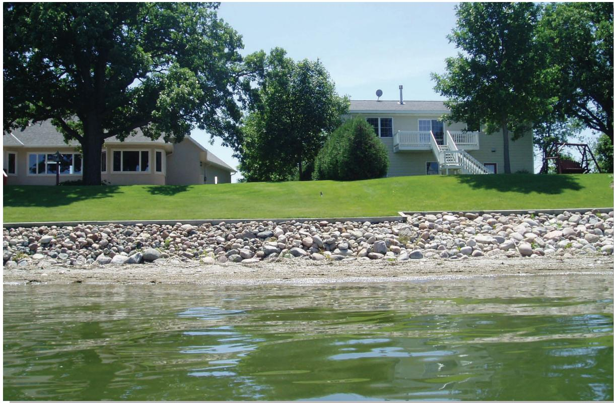
Figure 3. Sand/gravel giving way to riprap – recorded as RR.
