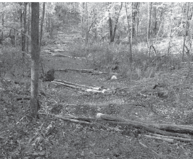
▲ This site illustrates an example of properly installed log water bars. Water bars divert water from forest roads and skid trails to reduce erosion. Implementation monitoring measures the use of such practices and provides the MFRC with information to improve harvest practices. Photo: MN DNR.
