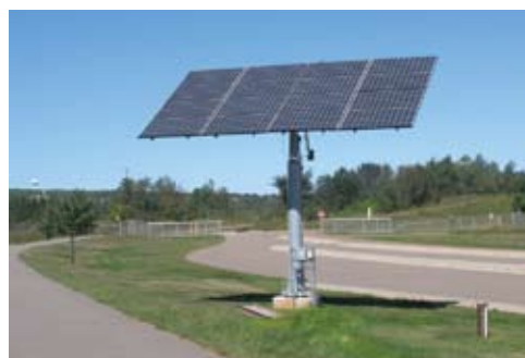
This photovoltaic array at the Iron Range OHV Recreation Area tracks the path of the sun, producing over 5,700 kWh per year.
