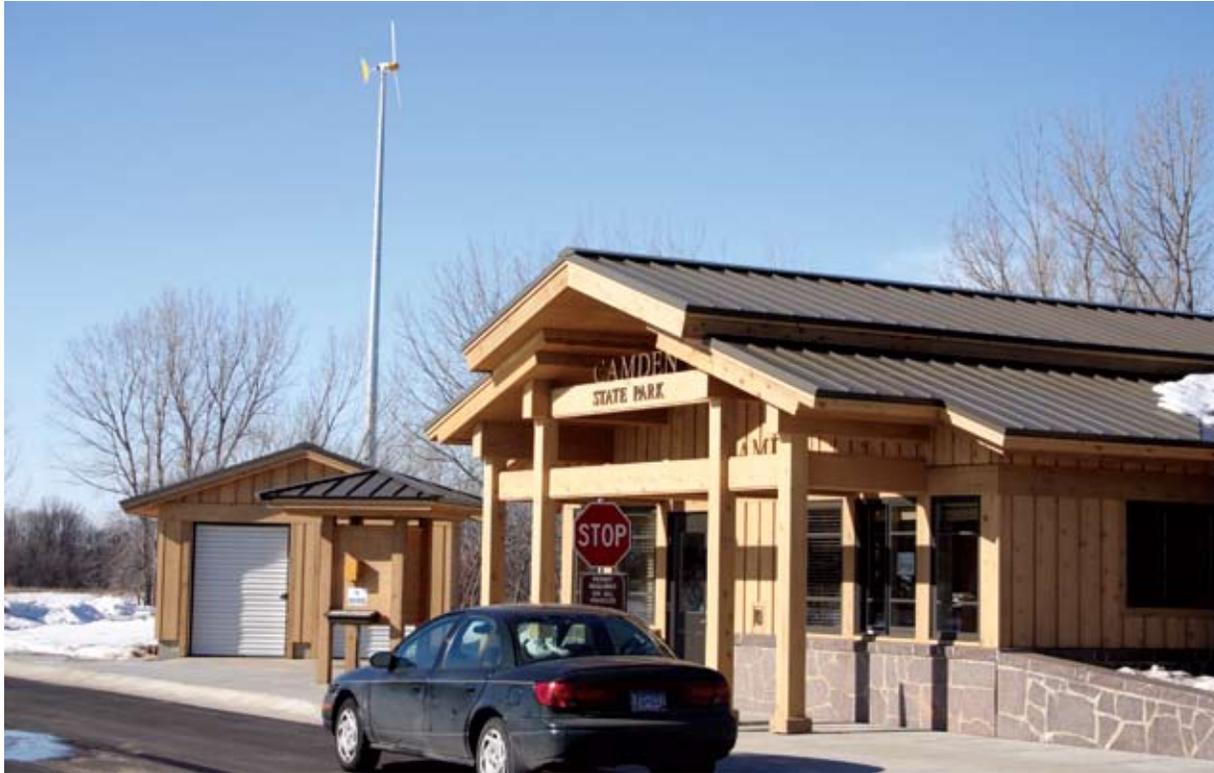
The Camden State Park contact station used the B3 Minnesota Sustainable Building Guidelines in its design, and includes a geothermal heating system and a 10 kW wind generator. The systems are sized to cover the energy needs of the building, making this DNR's first carbon neutral building.
