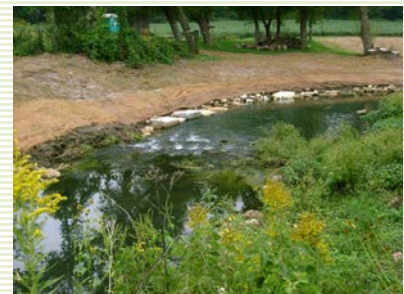
A before (above) and after(below) photo of Hay Creek, provided by Trout Unlimited, is taken before and after seeding, mulching and placement of erosion control blanket in 2010.
